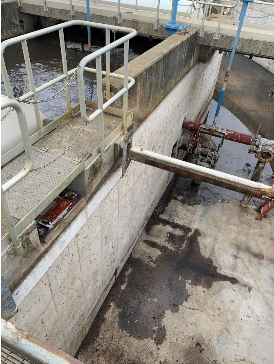
Photo #3: RAS Pipe (in red) with failed coating
