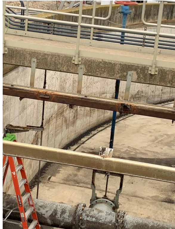
Photo #2: Beam rust at welds
