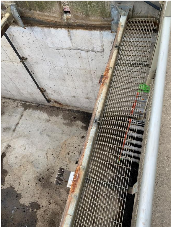
Photo #1: Beam rust at the welds
